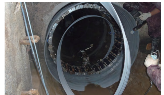
Restoration of aging sewerage pipes (SPR method)
