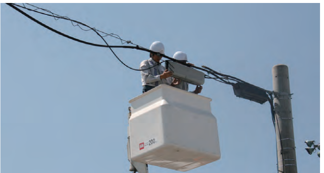
Work to connect optical fiber cables
