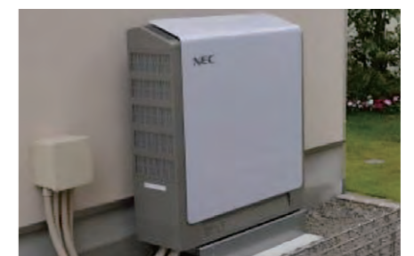
Electricity storage system for a freestanding house
