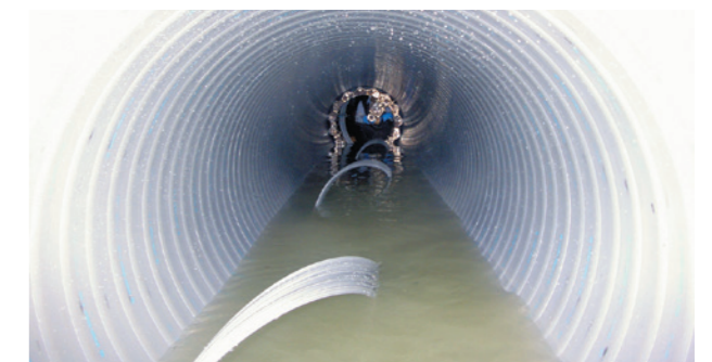
SPR method that allows construction to proceed amid flowing water
