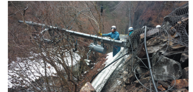
Recovery effort at a landslide site in Chichibu
