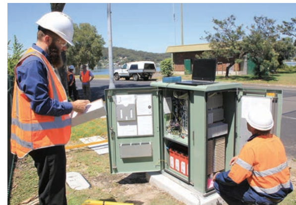
Connecting optical lines in Australia
