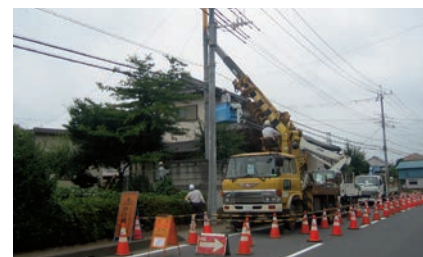
Replacing utility poles on privately owned land
