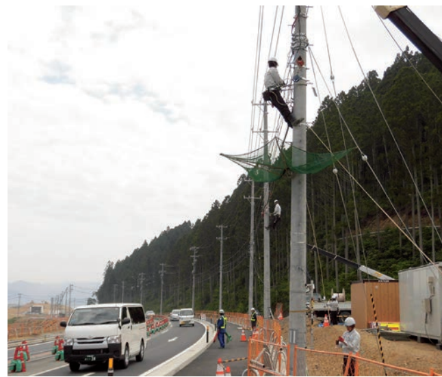
Stringing a cable
