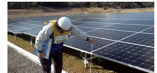
Quality inspection conducted by MIRAIT
