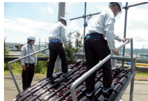
Training simulating a wet roof in rainy conditions
