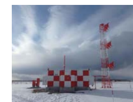
Glide path antenna showing the descent course (altitude)
