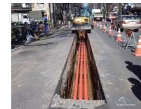
Construction Work to Lay Underground Cables (Electric Cable Multipurpose Underground Duct)
