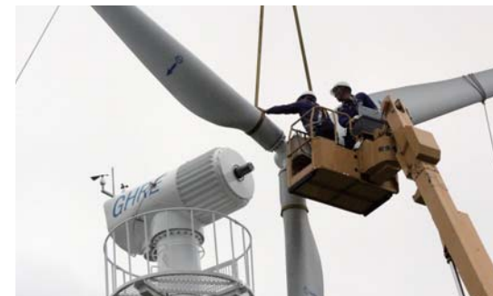
Attaching wind-power generator blades to the generating mechanism
