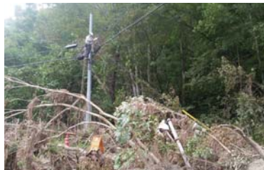
Emergency restoration construction in Iwaizumi-cho, Iwate Prefecture
