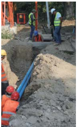
Optic fiber installation in Myanmar
