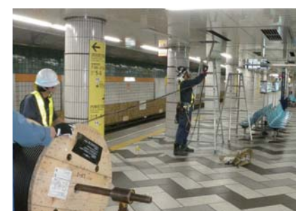
Construction of Dead Band Improvements Between Subway Stations
