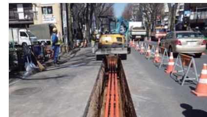
Construction Work to Lay Underground Cables (Electric Cable Multipurpose Underground Duct)
