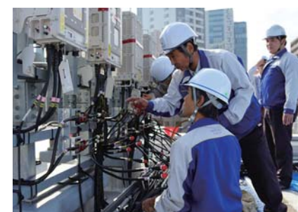
Construction of Wireless Base Stations
