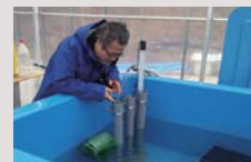
Water Quality Sensor Installed in the Water Tank
