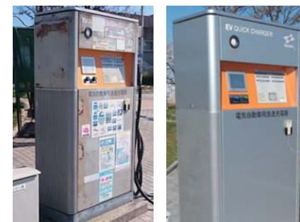
Repair of a rapid EV charging station with visible age degradation and rust using a lapping sheet
