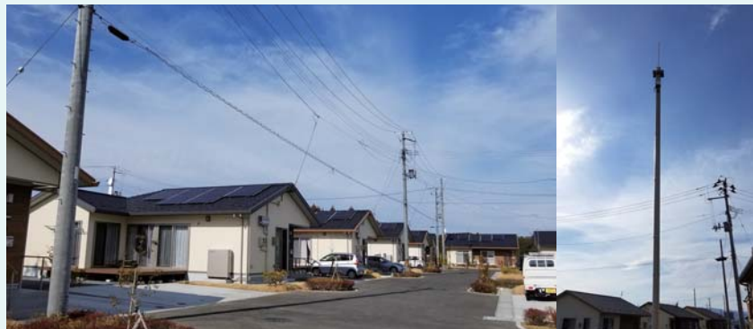
Left: Townscape of a Smart Community Right: LoRaWAN Gateway Pole
