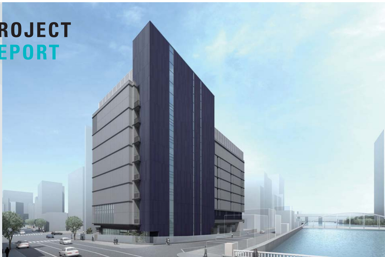
Exterior View of the 1st Osaka Data Center
