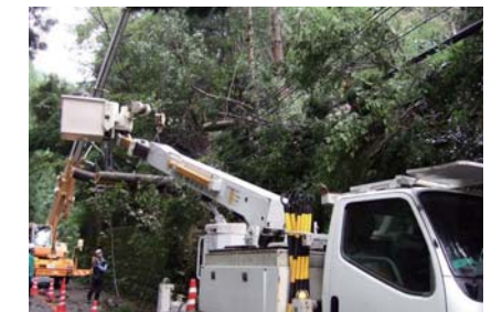
Recovery of the Aerial Communications Facility Stopped Due to Fallen Trees (Typhoon Jebi)
