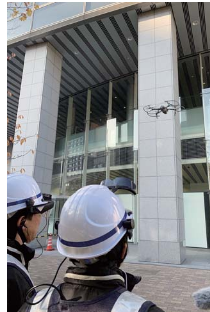
External building wall inspection using a drone and AR smart glasses
