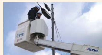
Students standing in the boom bucket of a bucket truck
