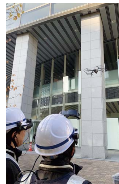
Building exterior wall inspection using drones and AR smart glasses
