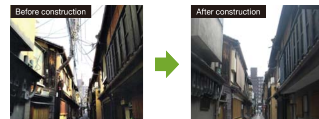
Construction to eliminate utility poles in Ponto-cho
