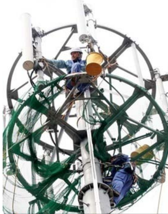
Attachment construction work of wireless base station for mobile phones (Miyagi)
