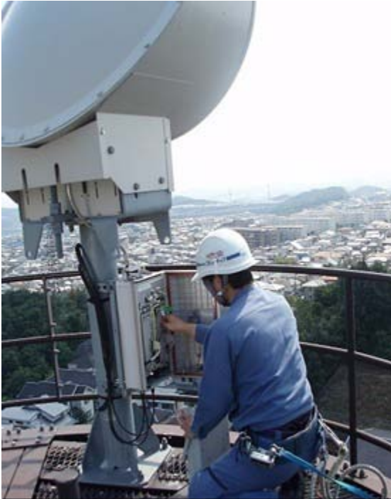
Maintenance and inspection of wireless base stations for mobile phones (Osaka)
