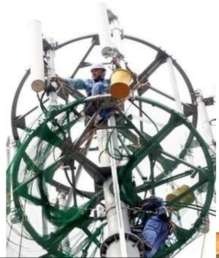
Attachment construction work of wireless base station for mobile phones
