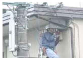
Laying optical fiber
