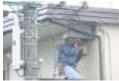
Laying optical fiber
