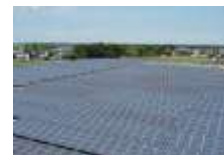
Building solar power plants
