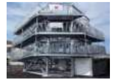
Construction of tsunami refuge towers
