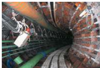
Construction of underground facilities
