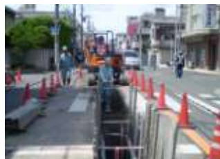
Work to lay underground conduits
