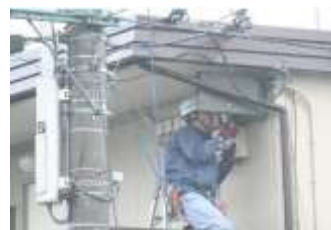
Laying optical fiber
