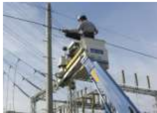
Setting up optical fiber
