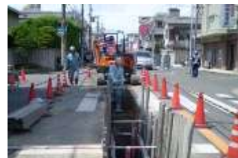
Work to lay underground conduits
