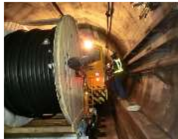
Work to resolve poor signal areas between subway stations
