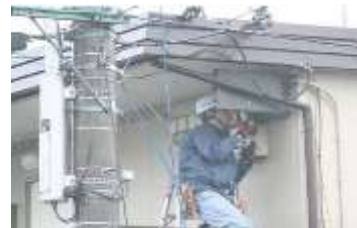
Laying optical fiber
