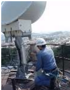
Maintenance inspections of wireless base stations
