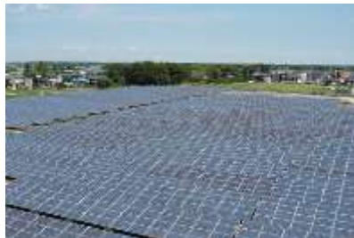
Building solar power plants
