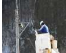
Optical cable connection work
