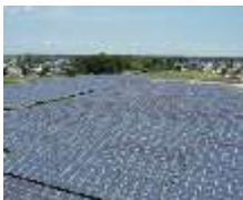
Solar power work
