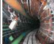
Construction of underground facilities
