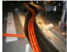
Laying power lines underground
