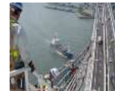
Repairing lighting equipment of highways
