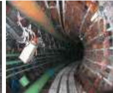
Construction of underground facilities
