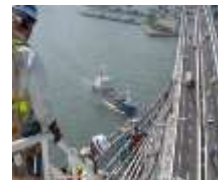
Repairing lighting equipment of highways
