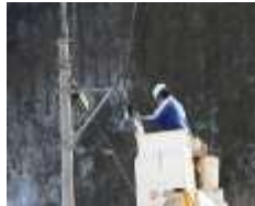
Optical cable connection work
