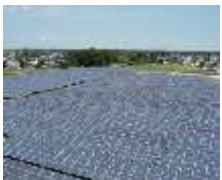
Solar power work
