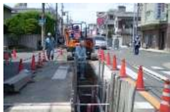
Work to lay underground conduits
