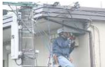
Laying optical fiber
