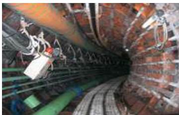
Construction of underground facilities
