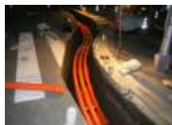
Laying power lines underground
