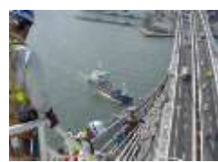
Repairing lighting equipment of highways
