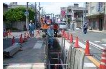
Work to lay underground conduits
