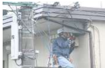
Laying optical fiber
