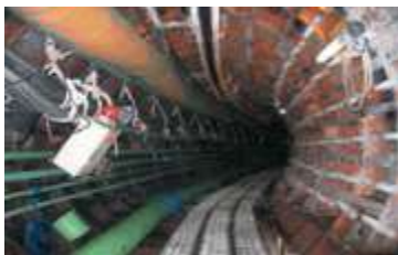
Construction of underground facilities
