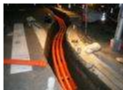
Laying power lines underground
