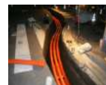
Laying of power lines underground
