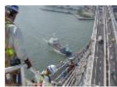
Repairing lighting equipment of highways
