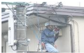
Laying optical fiber
