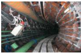
Construction of underground facilities
