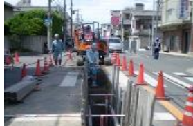
Work to lay underground conduits
