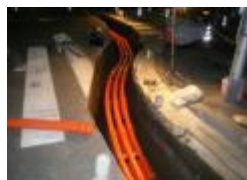
Laying power lines underground
