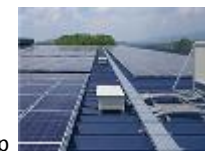
Solar power work
