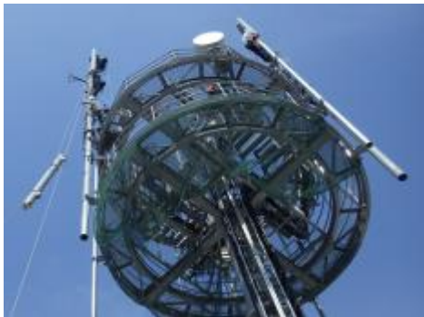
Wireless base station construction work
