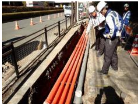
Laying of power lines underground
