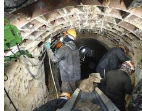
Civil engineering work (conduits)
