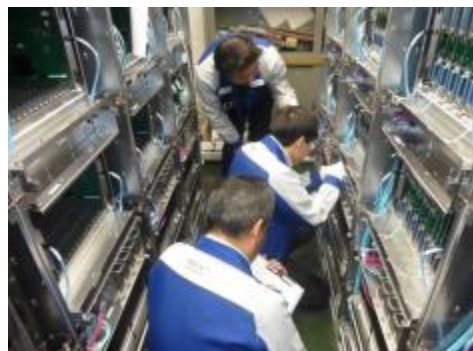
PBX renewal work
