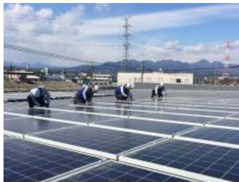
Solar power work
