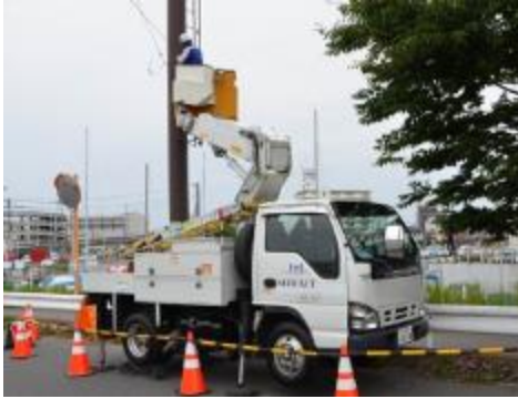
Cable connection work
