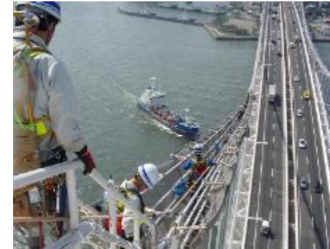
Repairing lighting equipment of highways
