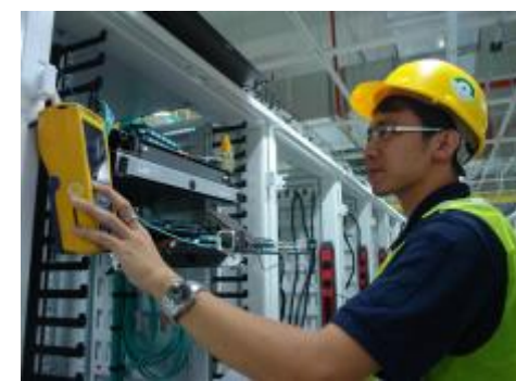
LAN cabling work (Lantrovision)
