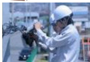
Optical line connection work
