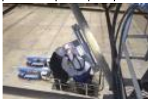
Construction of mobile base stations Work to improve reception quality
