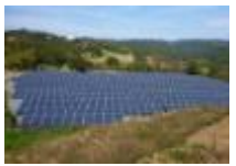
Solar power work
