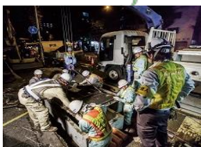
Work to lay power lines underground
