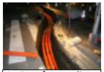
Laying of power lines underground
