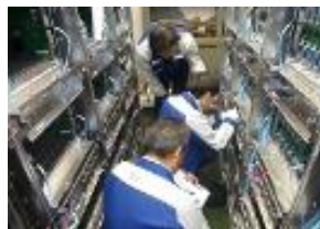
PBX installment work
