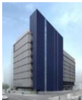
Large capacity, highly reliable data center in urban location
