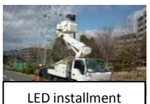
LED installment work
