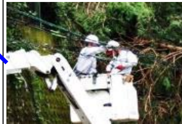
Disaster recovery work
