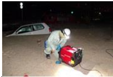
Supplying power to base stations
