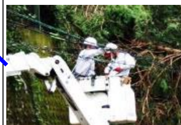
Disaster recovery work
