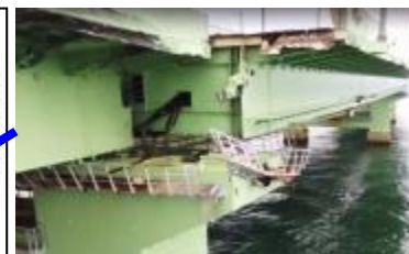
Damaged access bridge at Kansai Int'l Airport
