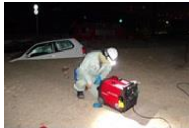
Supplying power to base stations
