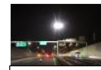
Lighting facilities in highways
