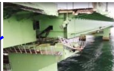
Damaged access bridge at Kansai Int'l Airport
