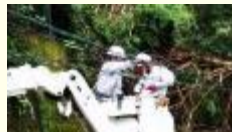
Rebuilding of utility poles and cables
