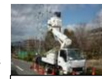
LED installment work
