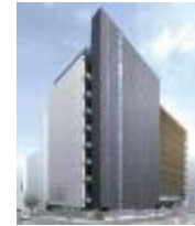
Osaka No.1 Data Center
