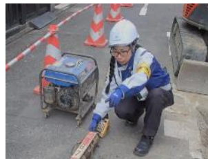
Water distribution pipe work (female engineer on-site)
