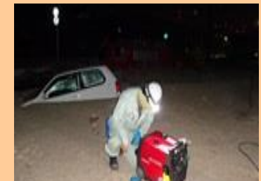
Recovery work for mobile base stations
