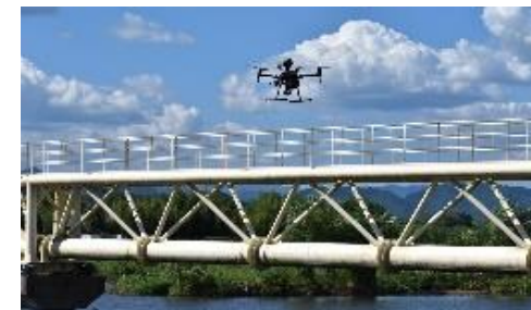
Water utility conduit inspection
