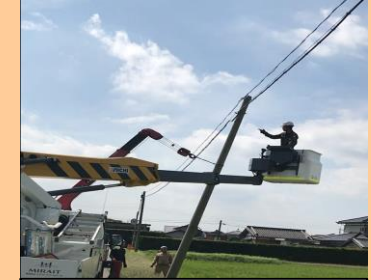
Rebuilding of utility poles and cables
