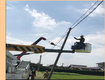
Rebuilding of utility poles and cables
