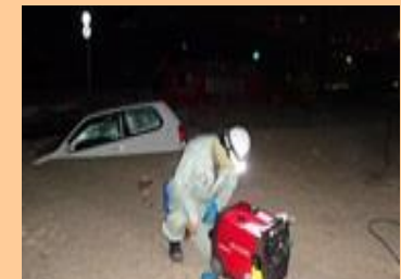
Recovery work for mobile base stations
