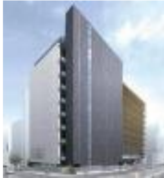
Osaka No.1 Data Center
