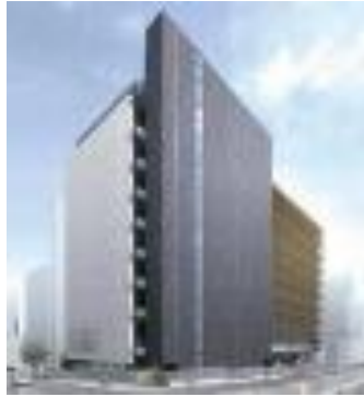
Osaka No.1 Data Center
