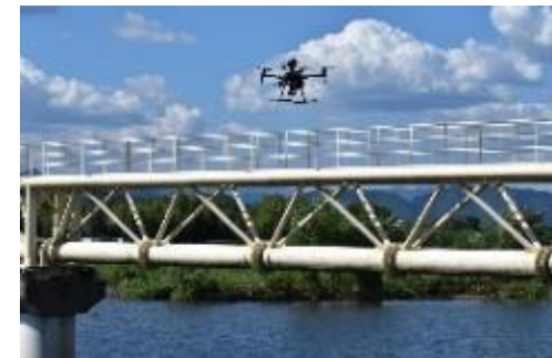
Water pipe bridge inspection
