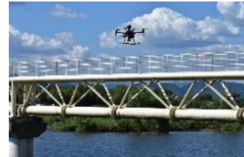
Water pipe bridge inspection
