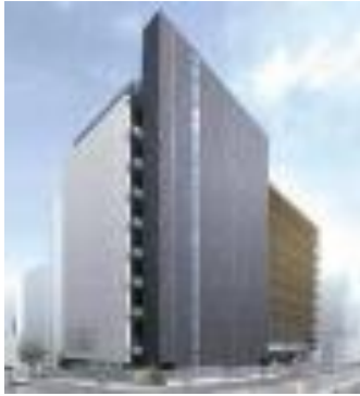
Osaka No.1 Data Center
