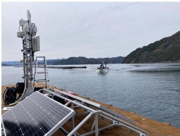
Solar panels for power supply
